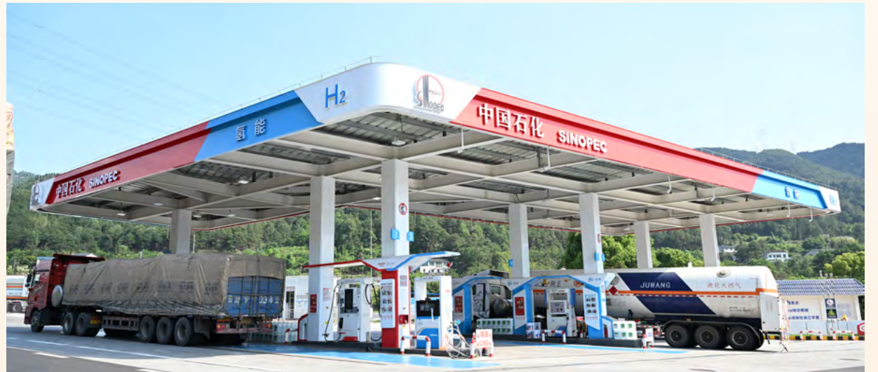
重庆公司“氢油气电”综合补能站 Chongqing subsidiary's "hydrogen, oil, gas, and electricity" comprehensive energy station
