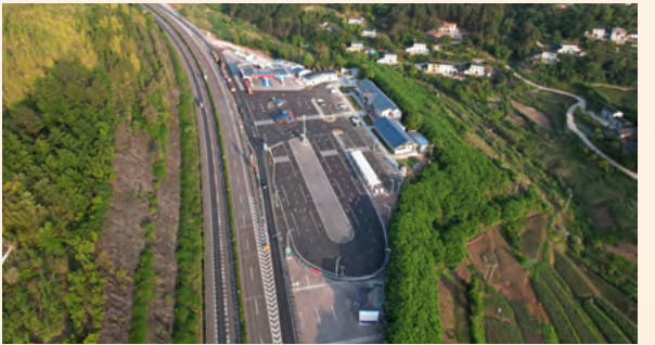
重庆公司黔渝高速赶水停车区俯拍图 Aerial view of Chongqing subsidiary's Ganshui Parking Area on Guizhou-Chongqing Expressway
